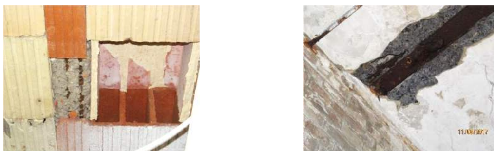
a) defects present to the underside of a hollow pot floor system b) defects present to the underside of a filler joist floor system
